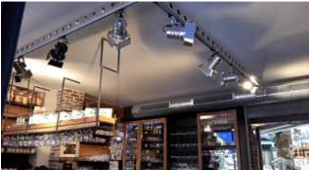
Trattoria Restaurant U-Match; Duct France
