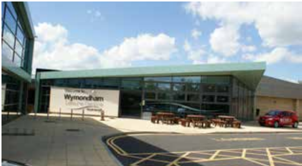
Wymondham Leisure Centre GMV5 Heat Recovery UK
